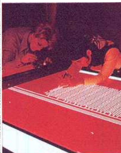
In Intel's early days, each layer of an integrated circuit design was drawn by hand, then transferred onto rubyolith. Operators such as the two women pictured here worked at light tables cutting each vector onto the red cellophane-like sheets. The rubyolith was then photostepped to the correct size and a mask was made.
