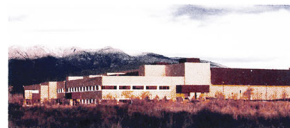
Fab 9 in Rio Rancho, New Mexico has Intel's largest clean room.
