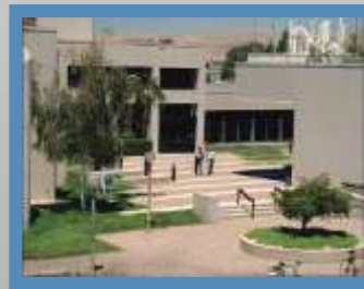
Transportation Energy Center Combustion Research Facility
