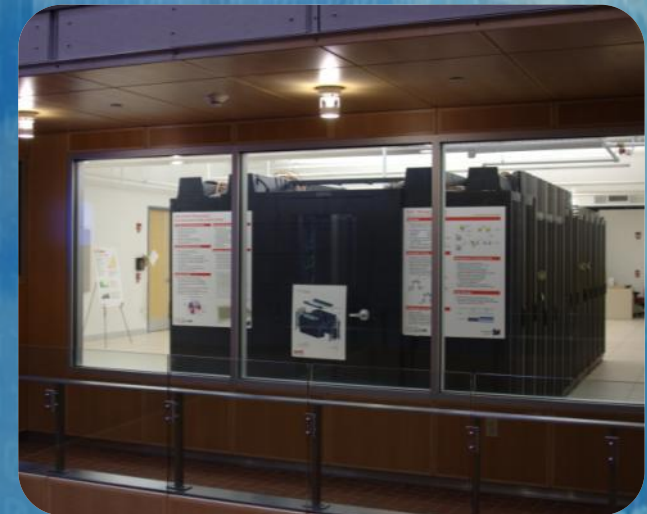
Data Center Observatory
