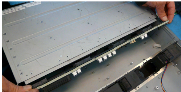
Figure 50. Pulling Back the Backplane and Lifting It Out of the Enclosure
