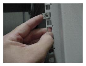
Figure 7. Attaching Clipnuts to the Rack
